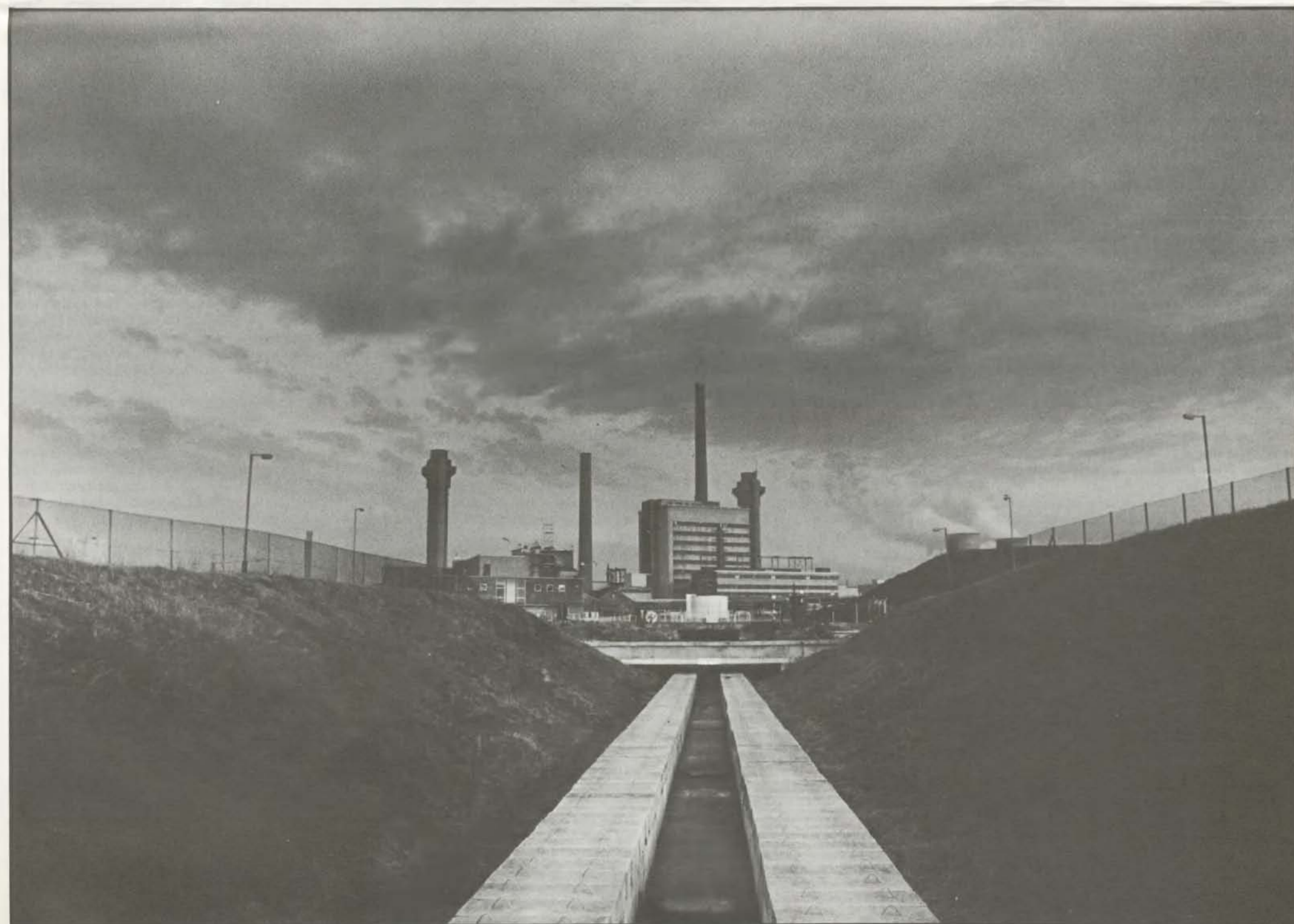
Pipes in concrete protection carrying radioactive water to the Irish Sea.
